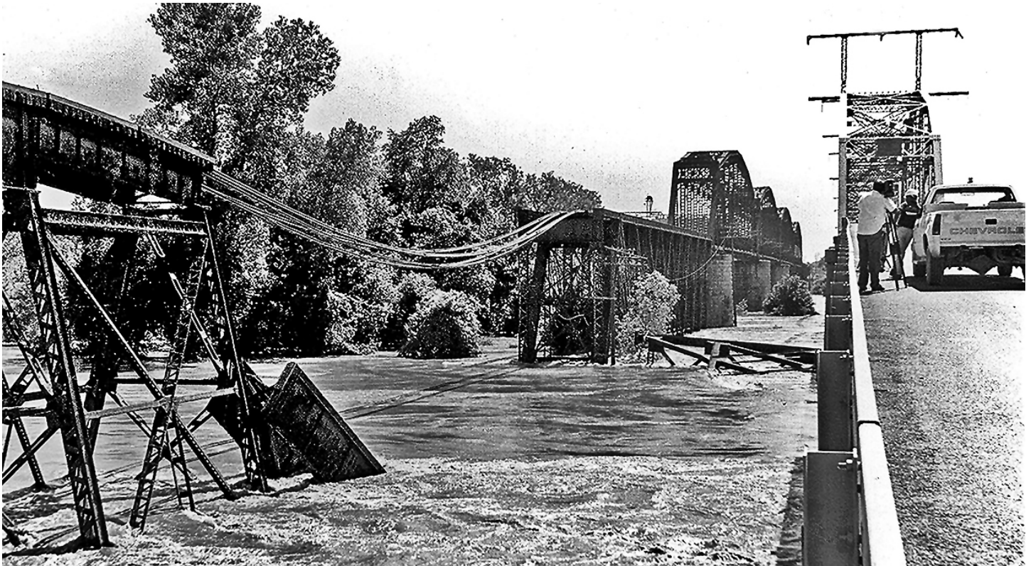
Flood waters destroyed a pier of the Kansas City Southern Railroad Bridge at Glasgow. The old highway bridge is at right. Photo by H. Denny Davis, Fayette Advertiser
