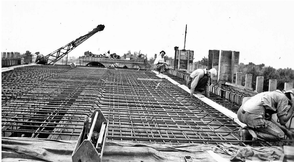
Construction of the viaduct began in 1939. Here workers are laying down the steel mesh substructure over which the concrete pavement was placed. Image courtesy MoDOT
