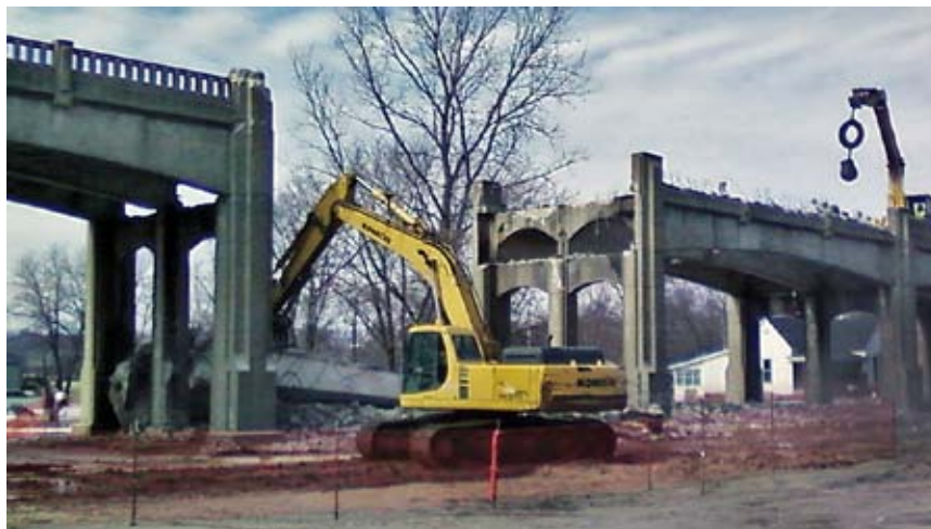
Demolition of the viaduct was completed in 2010 and took approximately three months. Traffic was temporarily routed around the work site. Photo by Jim Steele
